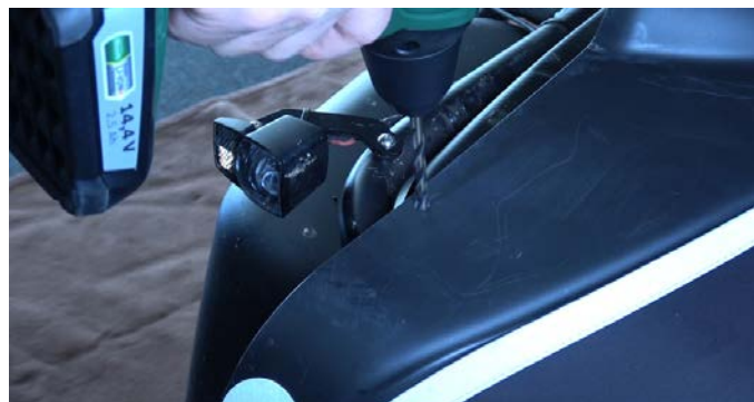
Fig. 6 Drilling the cable gland
